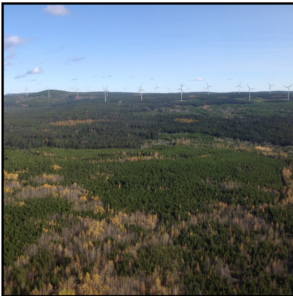
Windfarm in the middle of TRCF operating area.
