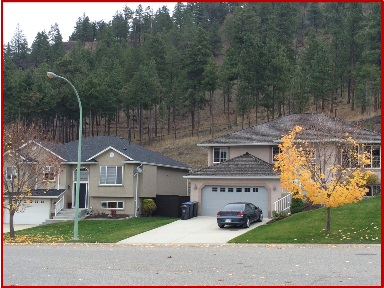
Figure 11. A fuel management treatment at Knox Mountain Park in Kelowna. Note the fire-resistant asphalt shingles on the house on the left and the cedar shake roof on the right.
