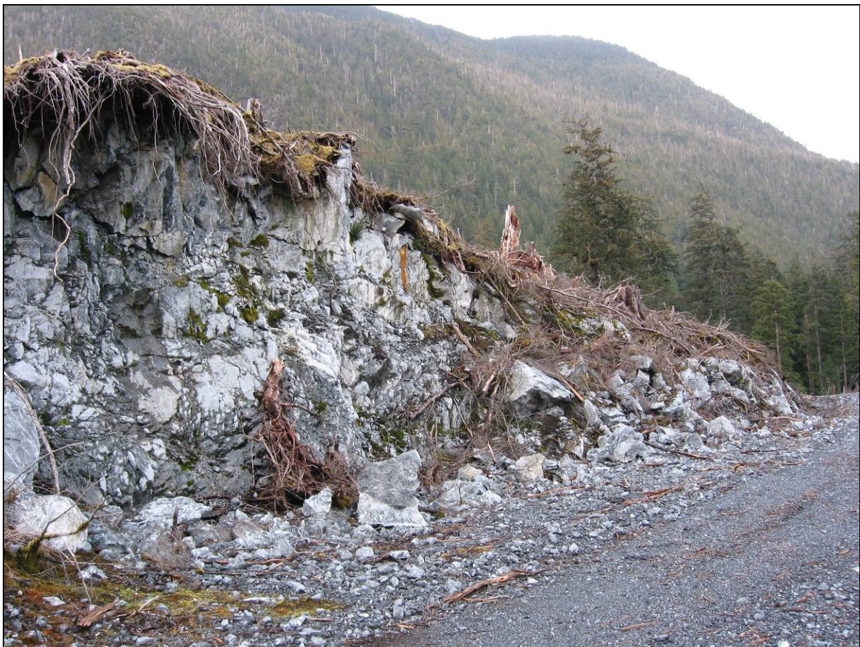
Figure 2 – Road building has special risks for karst, such as this irreparable damage from blasting
