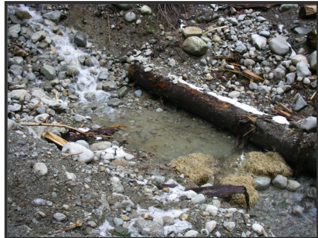
Photo 5. Opened log culvert where feeder creek crosses road deactivation.
