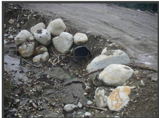
Photo 3. Upslope end of culvert.
