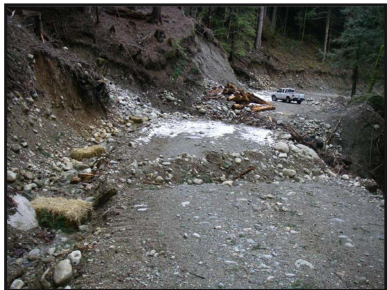
Photo 4. Hay bales in ditch leading to feeder creek during winter deactivation.
