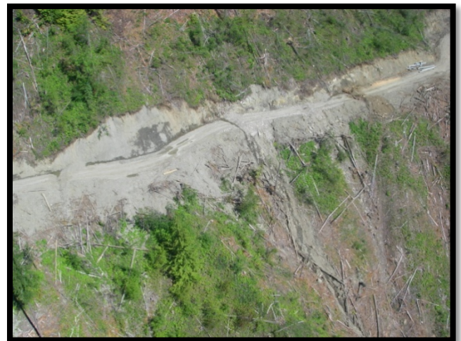
Engineered road construction causing erosion and sedimentation into a fish bearing stream.
