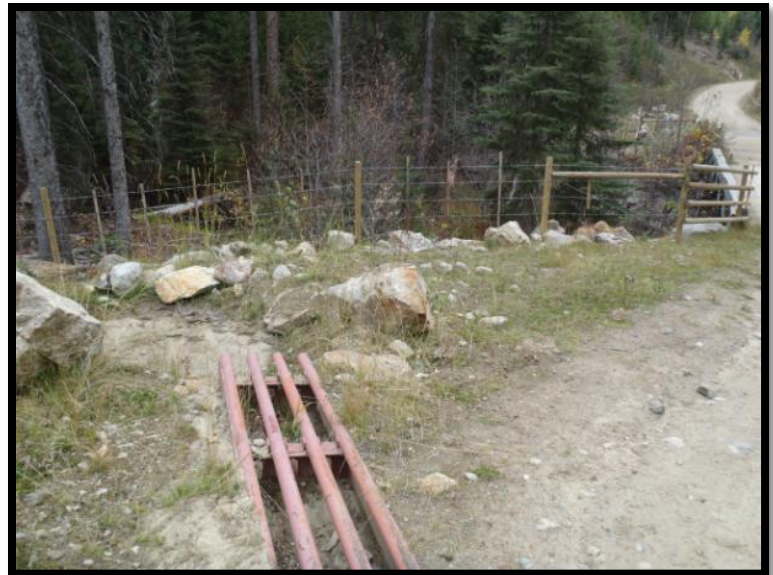
Figure 6 – Metal cross drain used to intercept sediment-laden road surface runoff and ditch water and direct it onto the forest floor away from the watercourse. Fencing and rip rap around the crossing exclude cattle from the watercourse.
