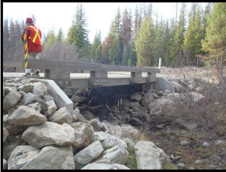
Figure 5 - Armouring with large rocks around the bridge protects the structural integrity of the bridge footings, and can sometimes deter cattle from accessing water at the crossing.
