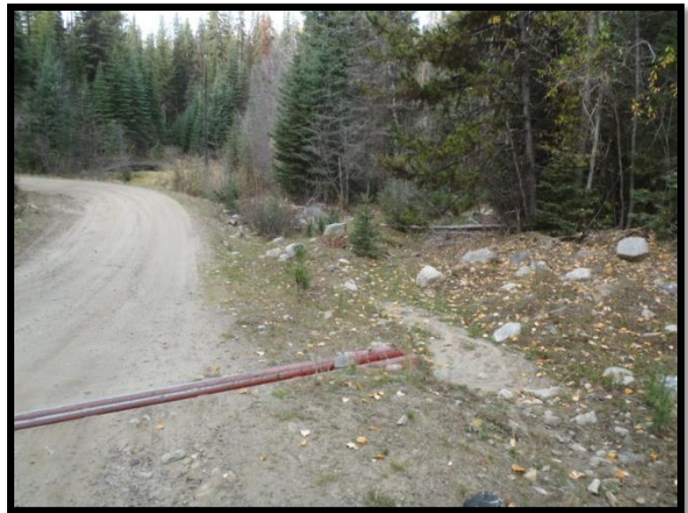
Figure 4 – Metal water-bar used to intercept and disperse road sediment across a BCTS FSR in the Oyama Creek watershed.
