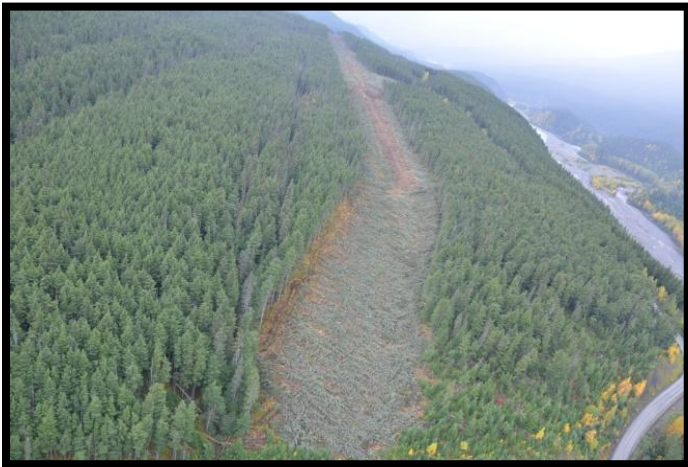
Hydro right-of-way construction.
