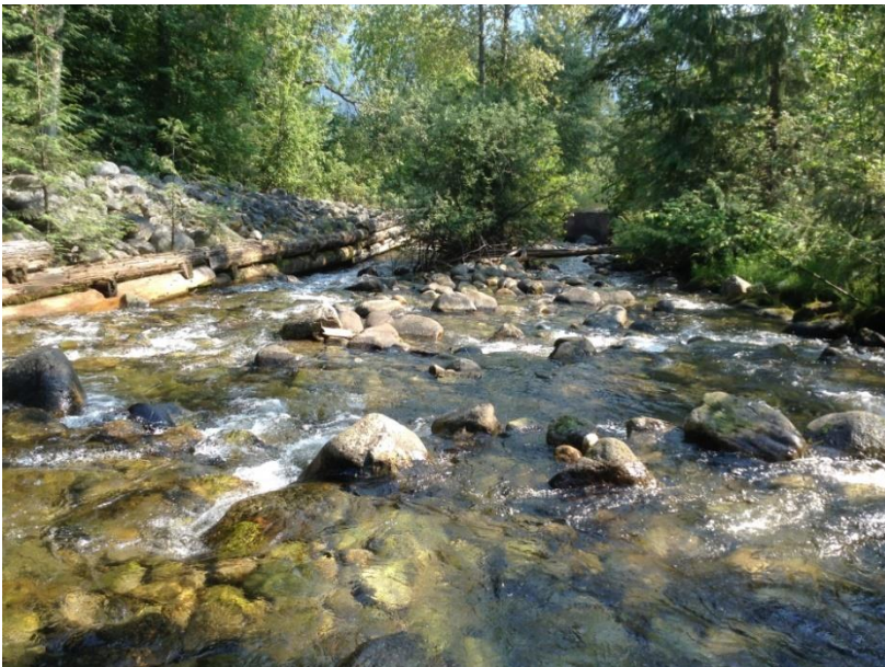
Photo 10. Looking downstream at 40 to 50 year old log crib wall along eastern bank that was built to contain Duhamel Creek during flood events. Additional material has been added to the top of this crib wall in the past few years.
