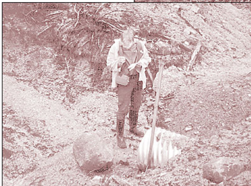
Culvert size and placement is assessed during an audit of road construction, maintenance and deactivation practices.
