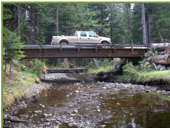
Figure 5. Bridge abutments set well back from the high water mark.
