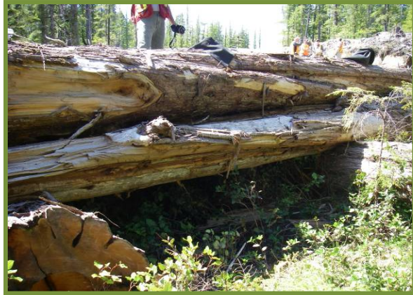
Figure 6. Open bottom structure (wood box culvert) on a small fish stream.
