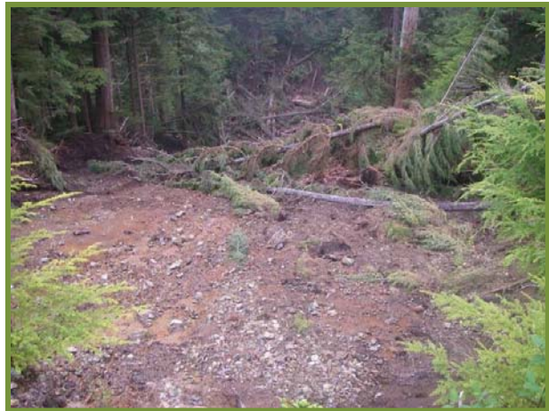
Figure 7. Landslide from an old road depositing into an important fish stream.
