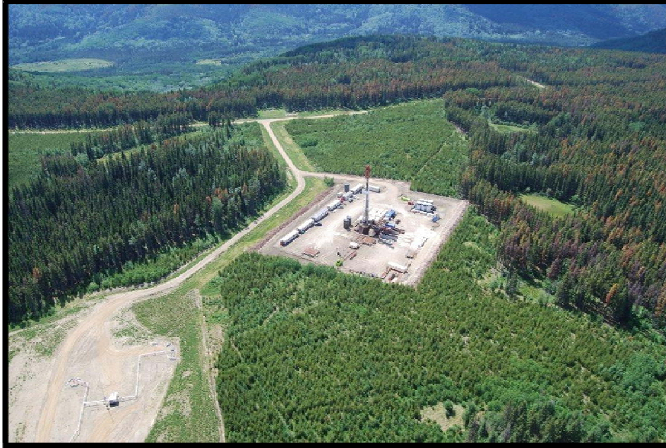
Figure 2. An active drill rig.
