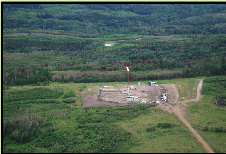
Figure 3. An active wellsite with a flare stack.
