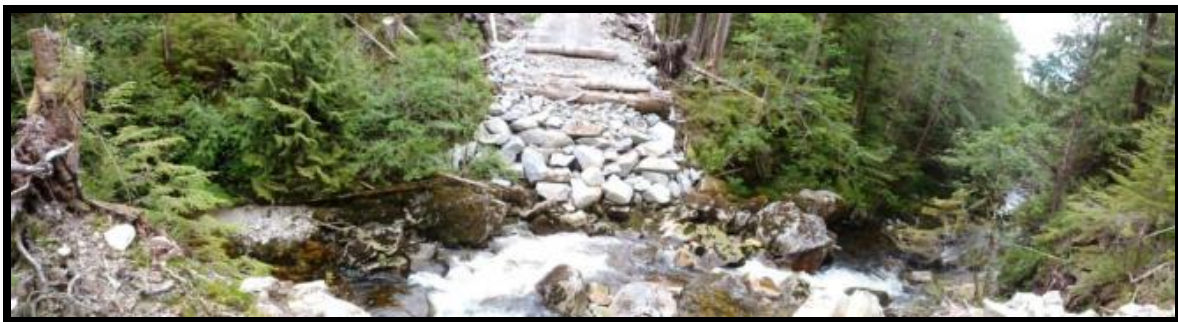
Deactivated bridge site on Naysash Creek.
