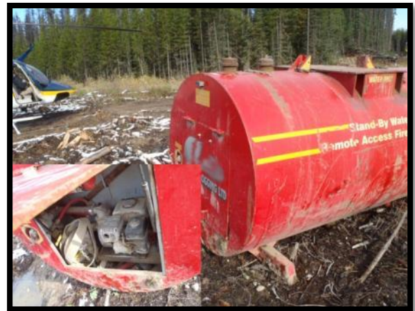
Water delivery system on an active logging site.
