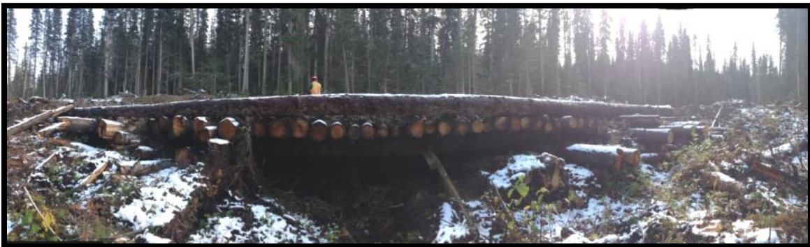
Overview of the log culvert installation.
