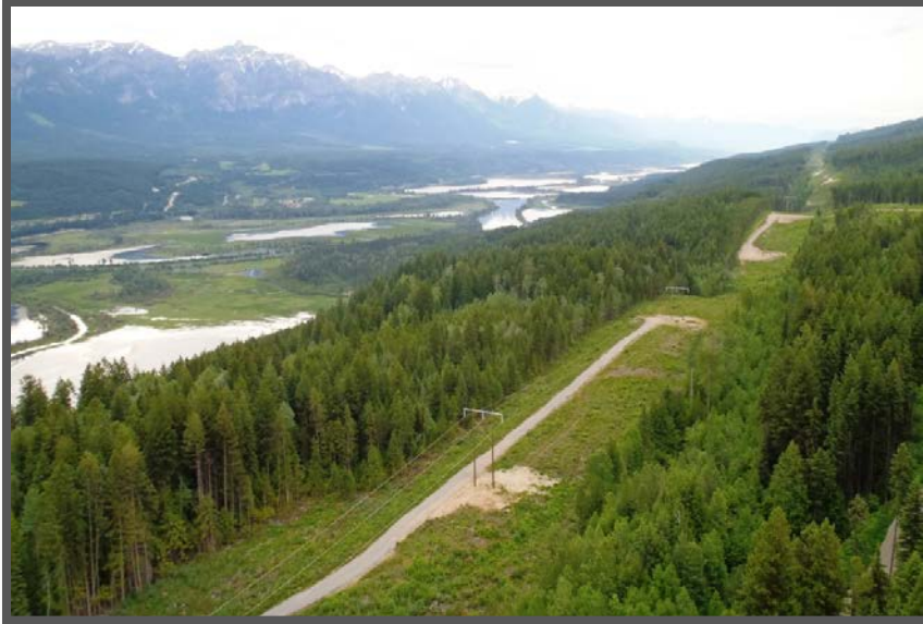
The Columbia Valley transmission line extending south towards Invermere: the low amount of residual slash depicted is typical of the slash levels retained along the entire length of the CVT project.
