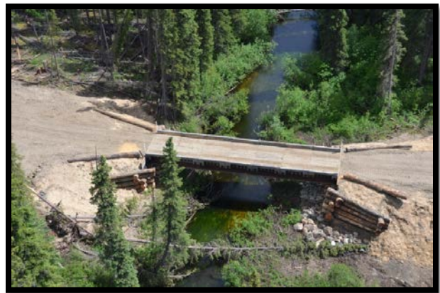
One of seven compliant bridges constructed by Carrier during the audit period.
