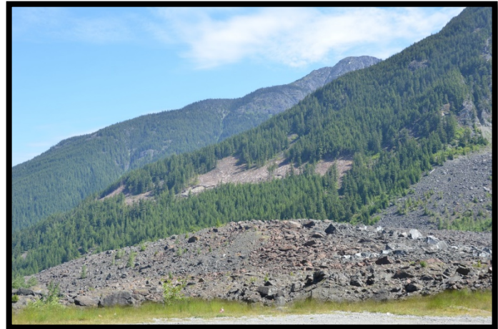
Cutblock as seen from the Hope Slide viewpoint. Rubble from the Hope Slide is visible in the foreground.
