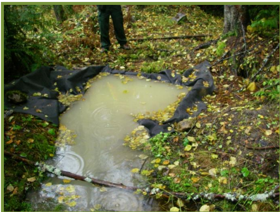
Sediment trap below Mounce Mainline. Note the suspended clay.
