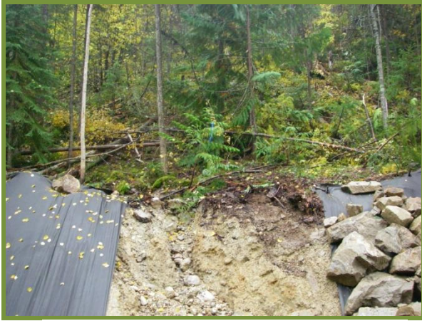
Subsurface flow at station 192.
