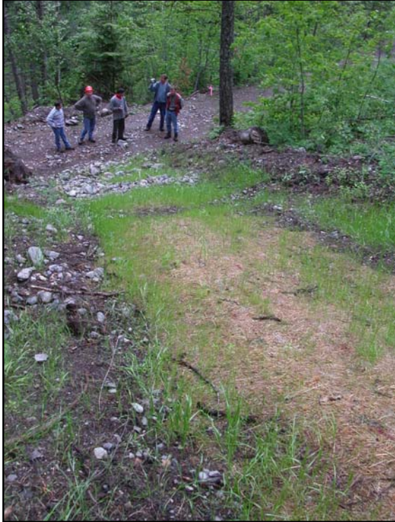
Erosion control blanket near Peterson Creek - McLure fire
