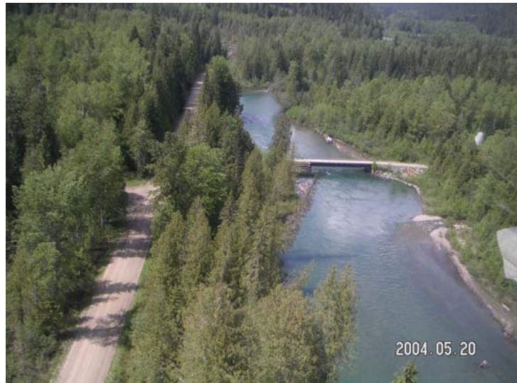
Figure 2 – Bridge in the Kootenay Lake Forest District
