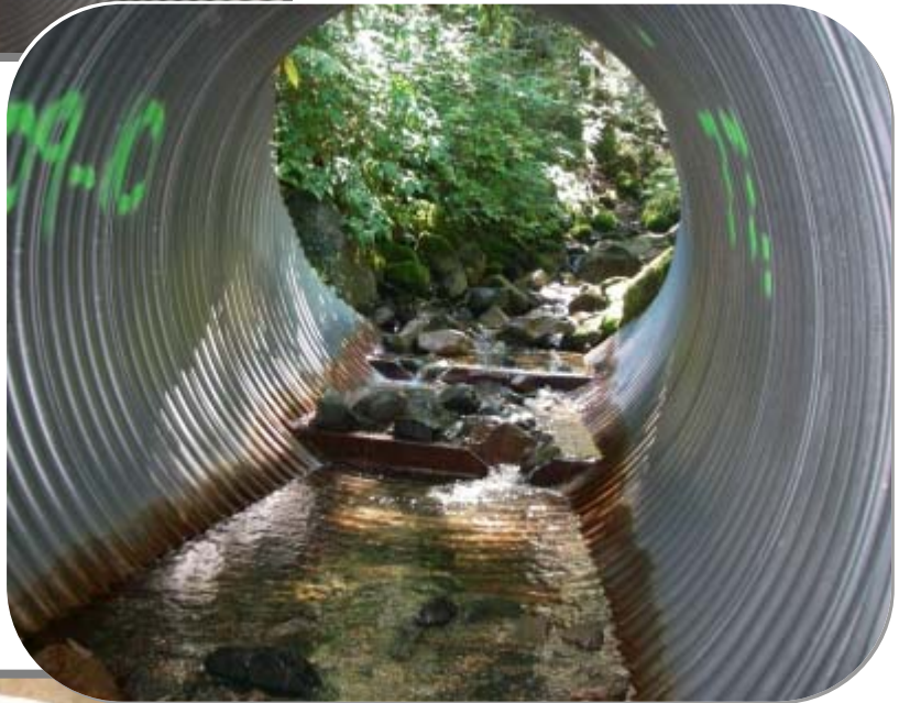
FIGURE 7. A round bottom culvert (CBS) with baffles to retain bed-load and create a more variable velocity profile.
