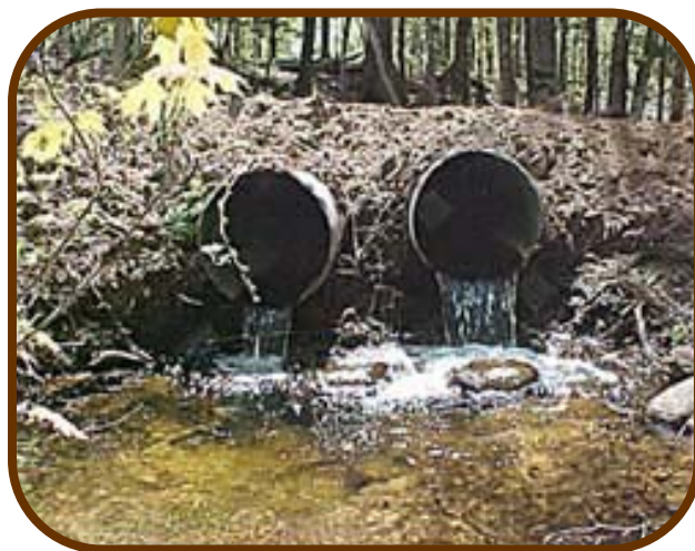
FIGURE 9. Elevated culvert outlets, with no plunge pool, prevent fish passage. Fish barrier score of 15.
