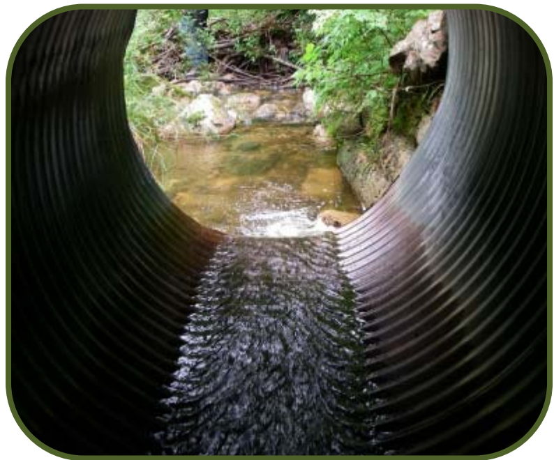
FIGURE 11. An example of a CBS culvert on an important habitat fish stream. The outlet drop and the length of the culvert, with no velocity refuge, is a partial impediment to fish passage.
