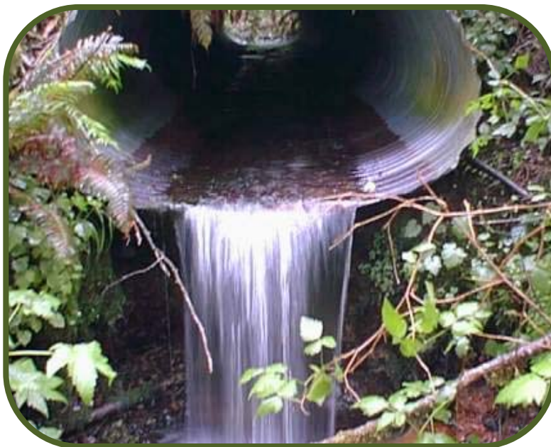
FIGURE 1. Outlet drops at culvert openings can impede or partially impede fish passage.
