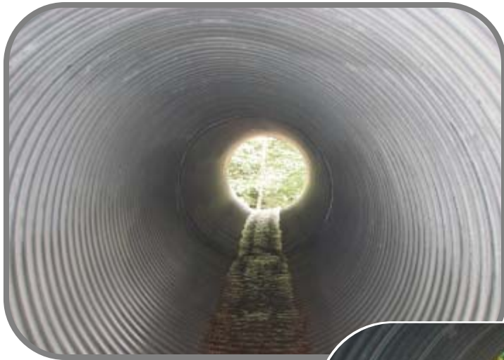
FIGURE 6. A round bottom culvert (CBS) with no embedded gravel.
