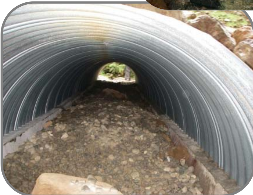
FIGURE 8. An elliptical arch culvert (OBS) retains the natural
