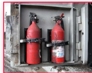
FIGURE 13. Fire extinguishers mounted on an excavator.
