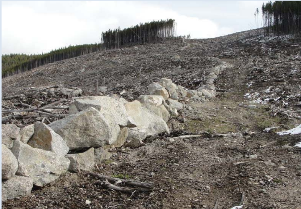
Figure 2. Case study #6. This one-kilometre long rock fence, which includes short sections of wire fence to permit wildlife passage, was constructed to mitigate the loss of a timbered natural range barrier. The rock fence was chosen as the preferred mitigation because underlying rocky material made a full-length wire fence unsuitable.
