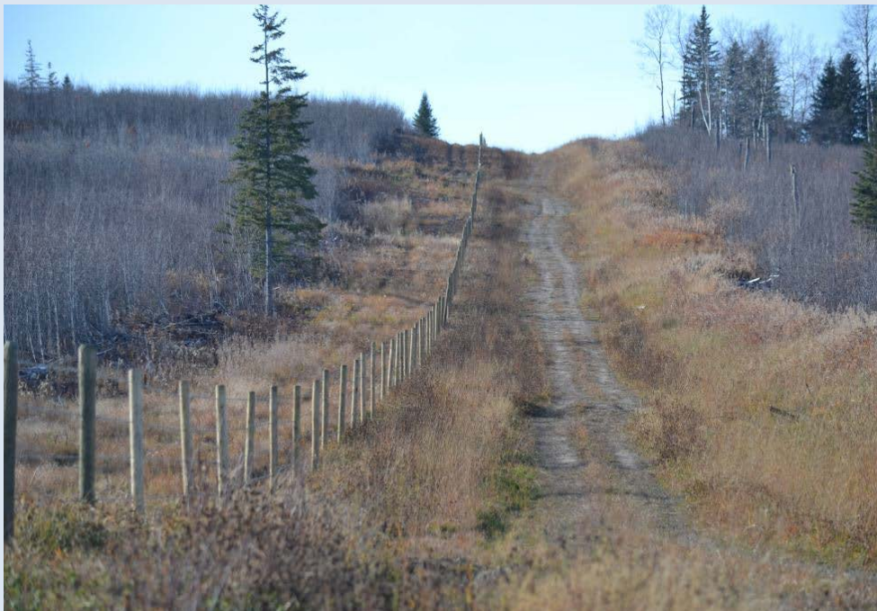
Figure 3. Case study #8. This wire fence was constructed to mitigate impacts to a natural range barrier. Wire fences are the most common approach used to mitigate impacts to natural range barriers.
