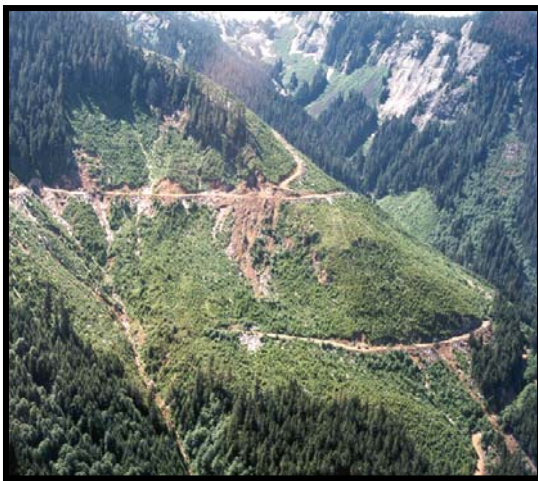
Old forestry roads can cause landslides. These old roads were seen during a Forest Practices Board audit.
