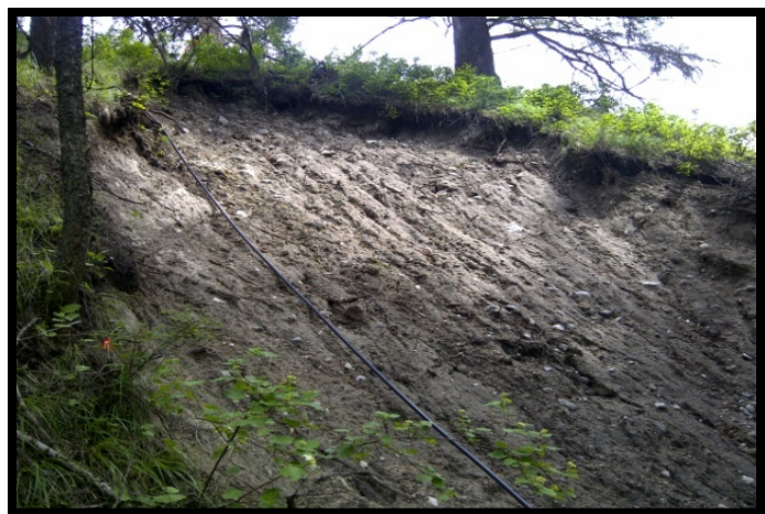
Photo 1. The slide and the outflow pipe running down to the creek.
