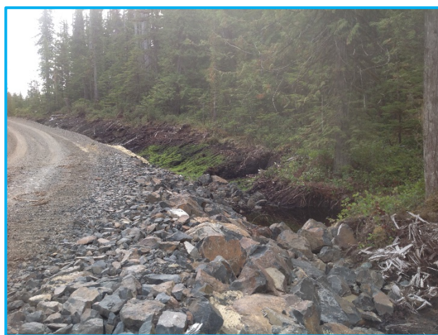
A fish stream approach where the road is capped with shot rock, sediment traps are installed and the road cut is seeded and mulched.
