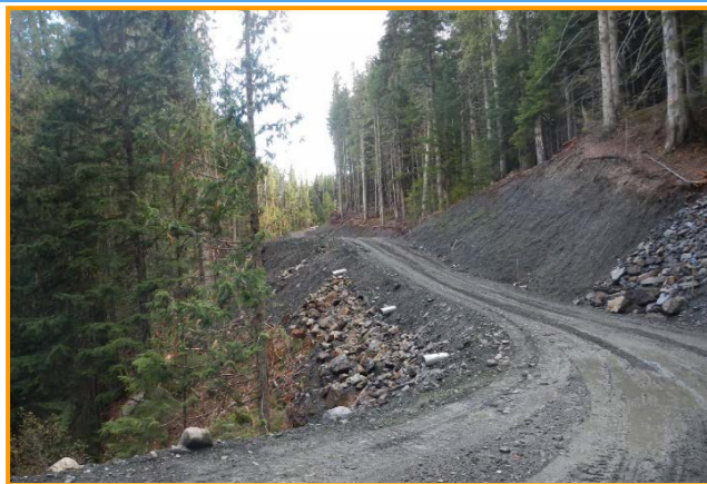
#2 – This is a road segment located through an area of imperfectly drained soils that required additional drainage structures and armoring of cutslopes and culvert outlets to avoid erosion. The work was well done.
