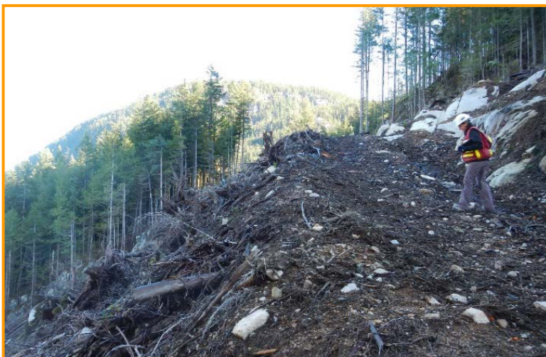
#4a – This is an example of professional designs completed incorporating terrain specialist’s recommendations. The terrain specialist recommended full bench construction with end haul from road stations 0+386 to 0+420.
