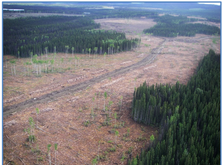
Typical terrain, harvesting and road construction.
