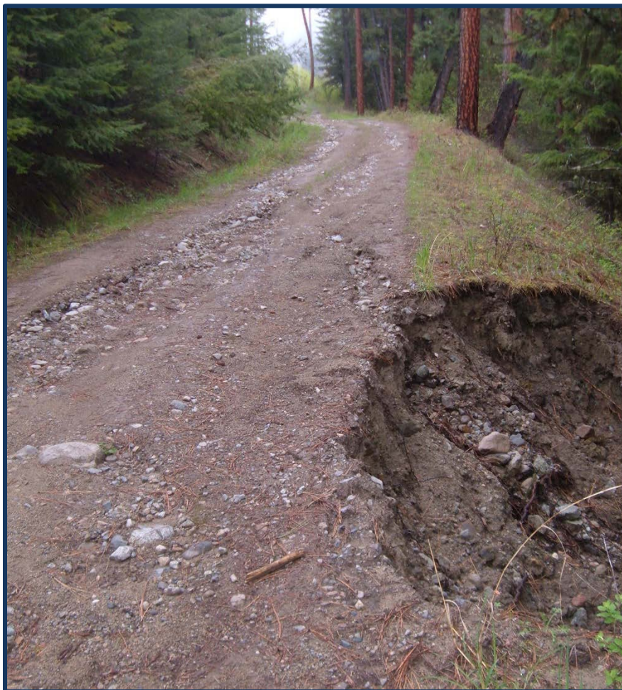
Figure 3. Surface run water saturated the road fill and caused a slump. Re-directed surface run water continued down slope and initiated a larger slide.
