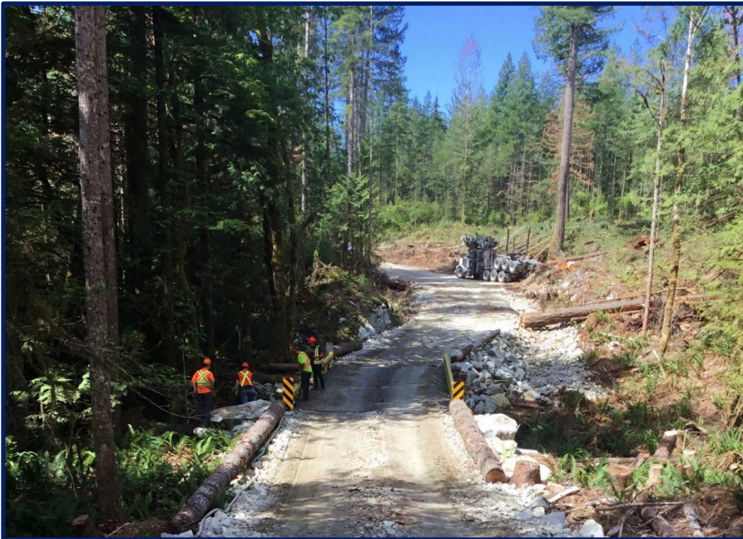
Auditors conducting a bridge inspection on the Sechelt Peninsula.
