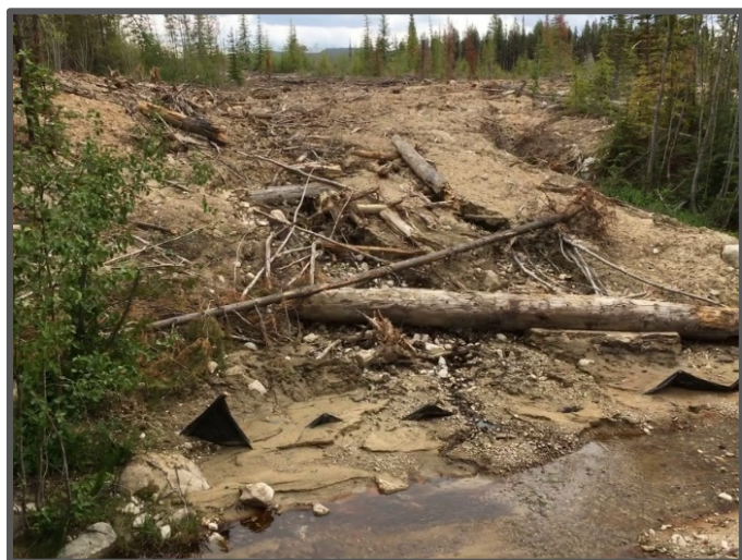
Figure 7. Photo shows where the sediment from the eroded ATV trail enters the main stream. The silt fence was put in place by the licensee during the removal of dirt in November 2017, and it was not installed to address sediment from the ATV trail.
