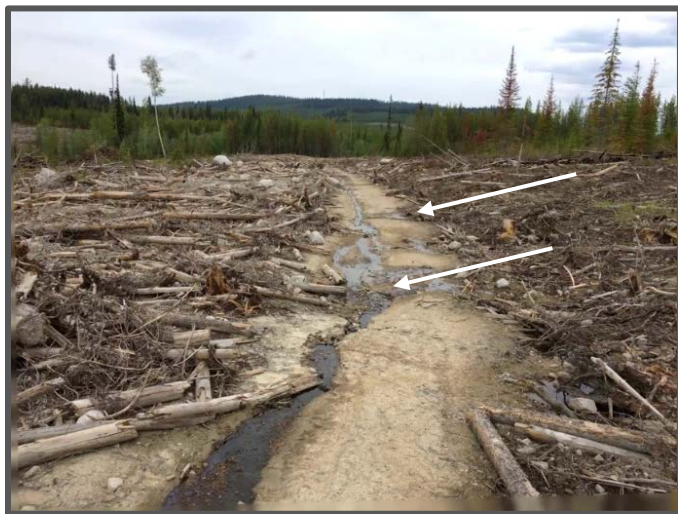
Figure 5. After harvesting, the licensee converted an in-block road to an ATV trail to provide access for replanting. During the 2018 snowmelt, this trail intercepted surface flows (see arrows) which were directed towards the main stream crossing.
