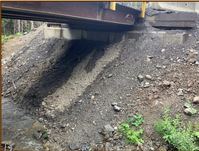
This stream bank is not armoured with rock and sediment is being introduced to the stream.
