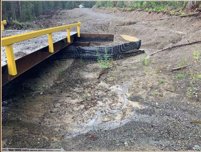
This crossing is contributing significant amounts of sediments to this fish-bearing (S4) stream.
