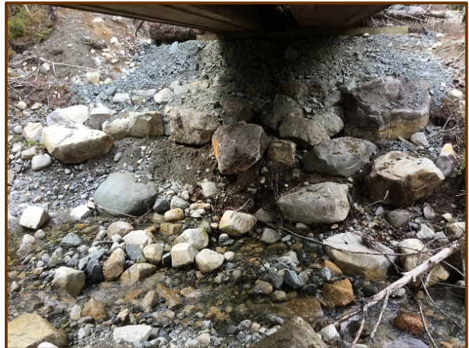
Inadequate armouring of the bank. Rock is not properly keyed in to withstand the stream flow and to retain the fill.
