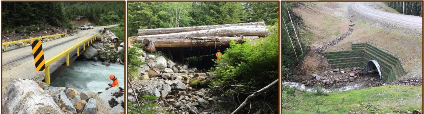
Three examples of crossings (from left to right): 27-metre steel girder bridge, log stringer bridge, and an engineered open-bottomed arch culvert.
