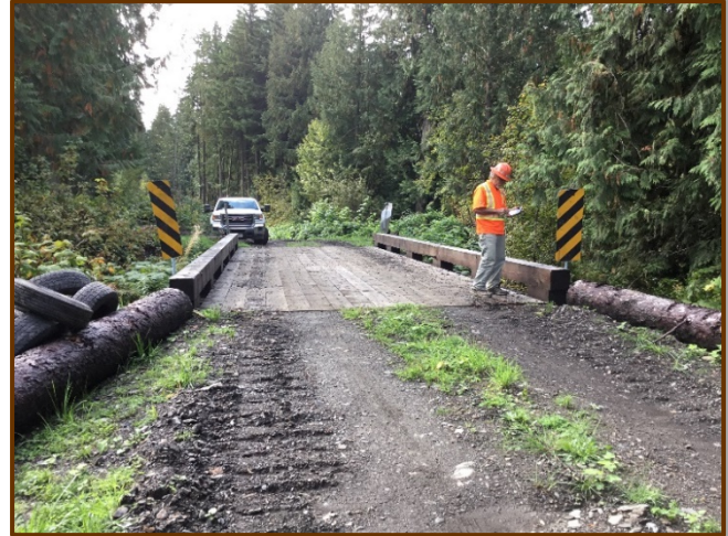
This 12-metre portable steel girder bridge with a timber deck sitting on double log sill abutments is a simple crossing.
