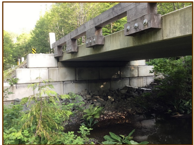
This 12-metre permanent pre-cast concrete girder bridge is designed to accommodate the peak flow expected in 100 years (Q100).
