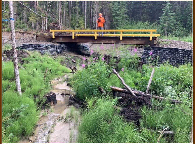
This crossing is contributing significant amounts of sediments to this fish-bearing (S4) stream.
