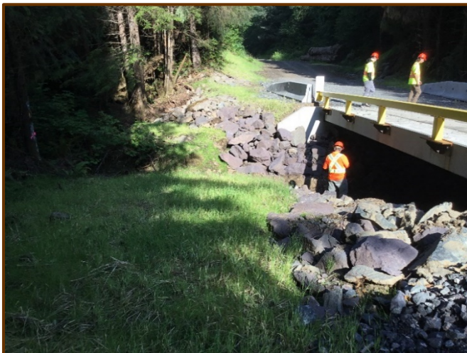
These banks are well armoured and disturbed areas have been seeded with grass to minimize sedimentation.
