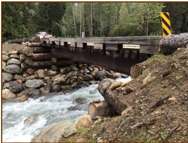
This 15.24-metre bridge was designed to accommodate the peak flow expected in 50 years (Q50). It will remain in place for up to 15 years.
