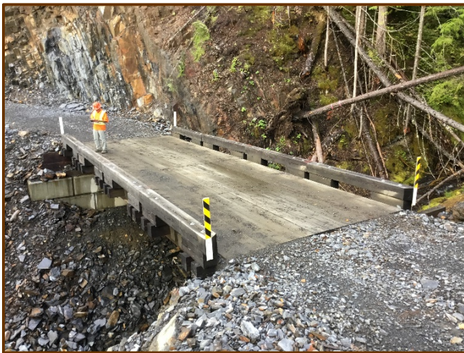
A 12-metre steel girder bridge with timber deck. The substructure of this bridge required extensive engineering expertise to determine the design bearing capacities, as well as the safety and stability of approach excavations. This is a complex crossing.
