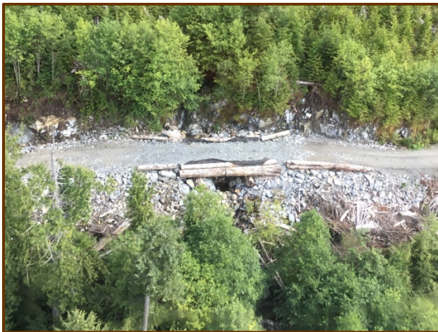
A wood box culvert. This is not a log stringer bridge because the span is less than six metres.
