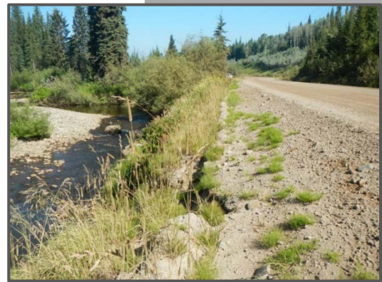
In some areas, the Morice-Owen Forest Service Road is located immediately adjacent to Owen Creek—a high value fish-stream. Sediment from the road directly enters the stream. In these areas, the riparian buffers have also been impacted.
