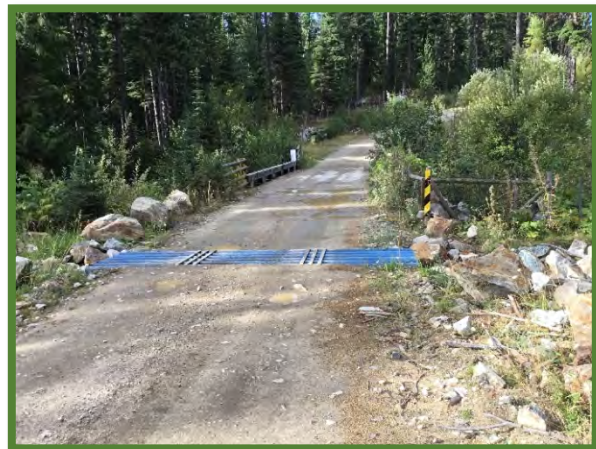
Range use is common in the Okanagan TSA. The maintenance of cattle guards and drift fences are necessary to control cattle movement.
