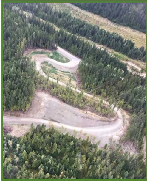
South Fork FSR was re-constructed to stabilize the road.
