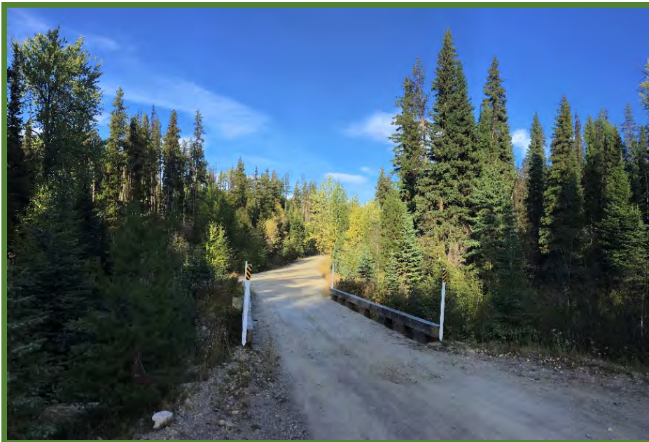
A typical FSR and major structure located near Peachland.
