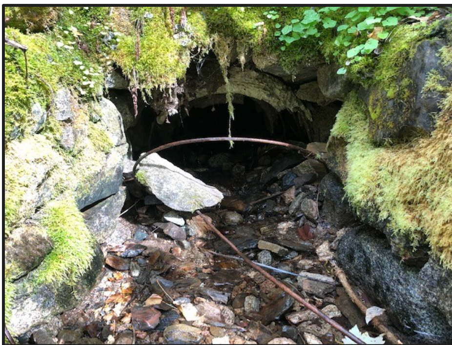
Figure 3. The old culvert replaced by Interfor on the small unnamed tributary stream.
