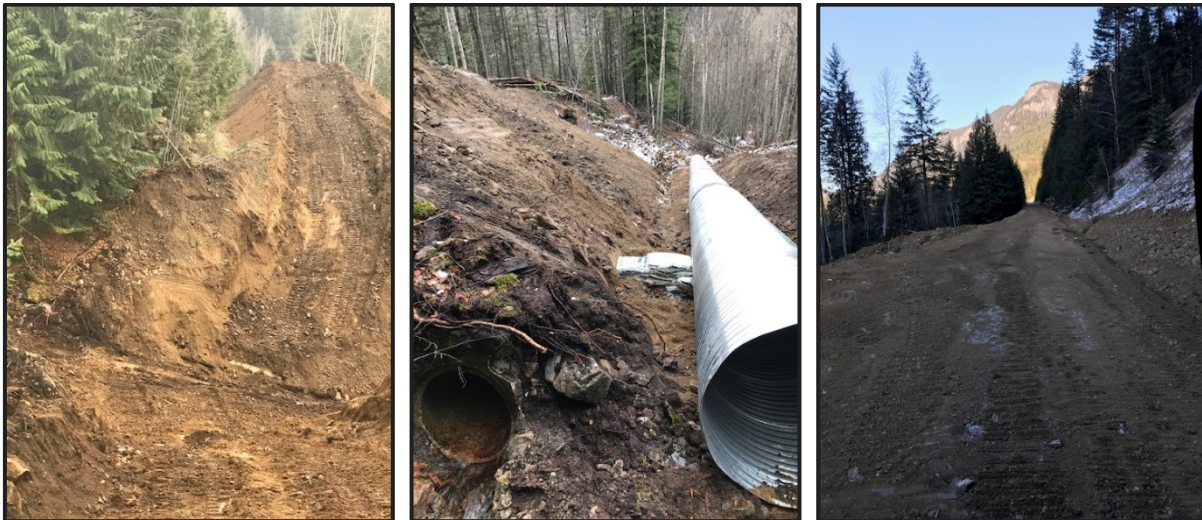
Figure 4. The culvert replacement site - during excavation, culvert placement, and final grade.
