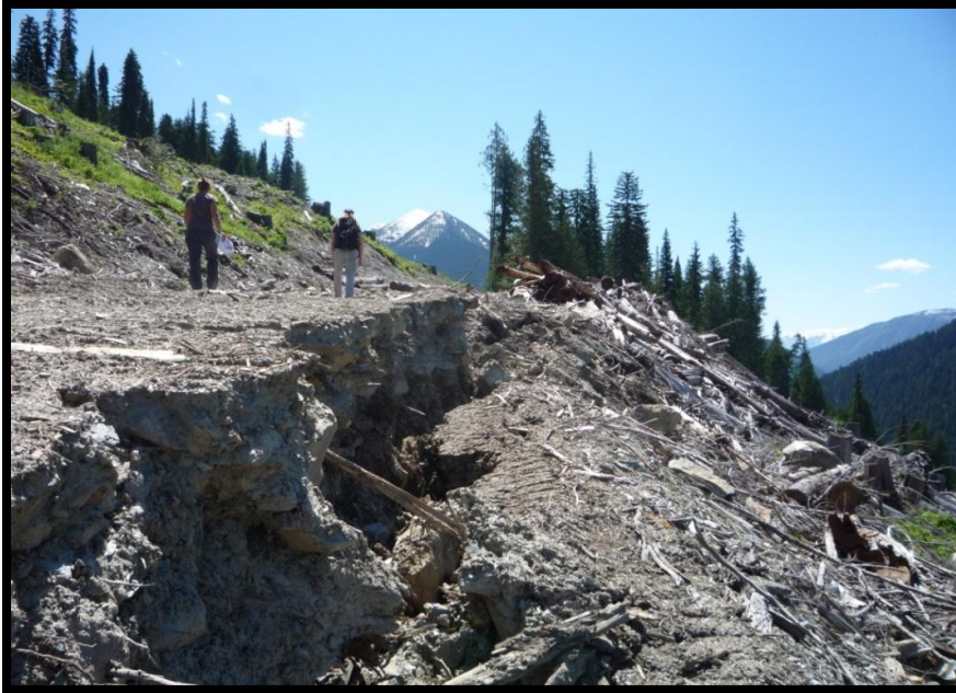
Poor road construction - failure of a 3-year old road prism. Note excessive organics in fill.
