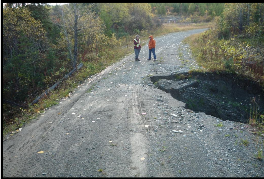
Road maintenance - failure of a road prism. Road under permit but considered a wilderness road. Structural integrity of the road prism has not been maintained, impacting a fish stream, therefore this is non compliant. Note the recent vehicle tire marks on this road.
