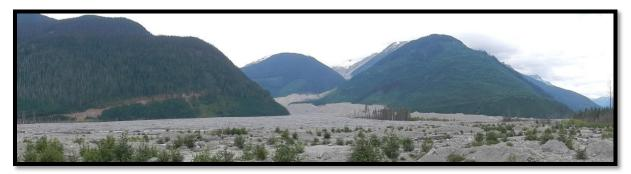
Debris from the Meager Creek landslide fills the Lillooet River. The landslide started at Capricorn Creek (centre-top), flowed down into Meager Creek (centre of photo) and then out into the Lillooet River (foreground.). Pebble Creek's new road accessing the Meager operating area is visible on the left hillside.
