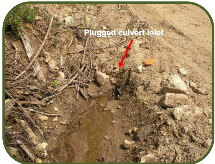
An example of a plugged culvert.
