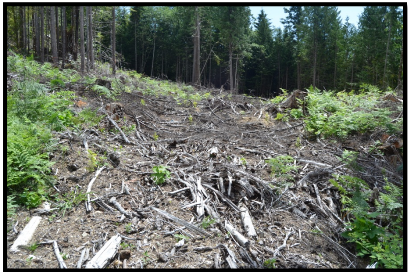
K3F - Temporary access structure within a recent cutblock showing rehabilitation of structure and planting when harvesting completed.
