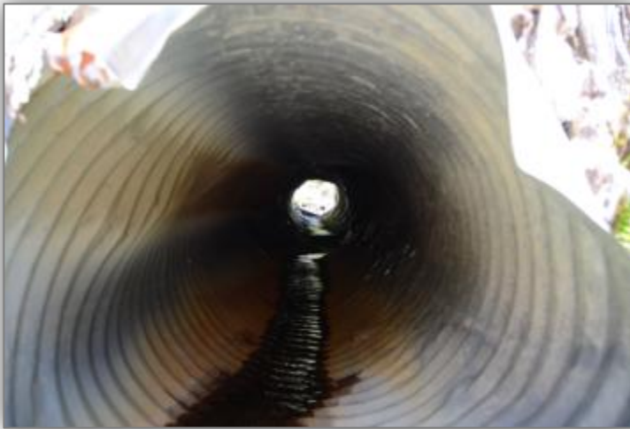
Looking through a functioning culvert on a spur road built to access timber on Woodlot 1903.
