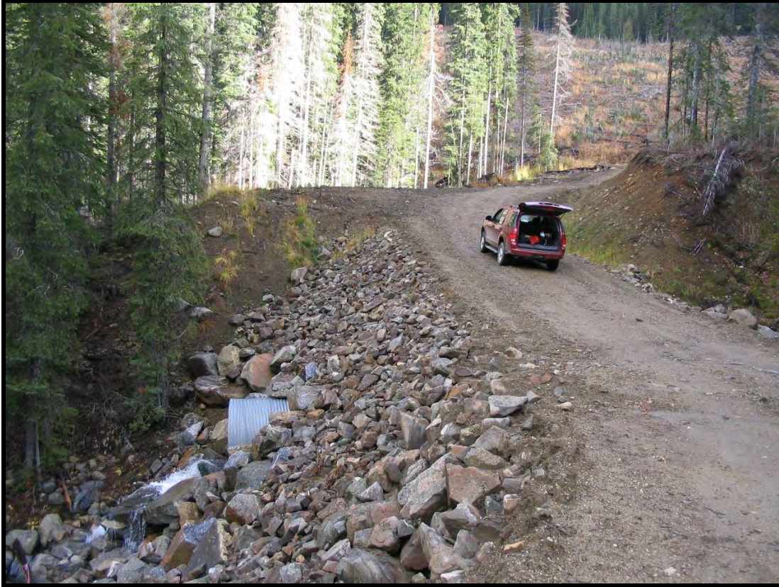
Figure 4. Well-stabilized road fill and culvert in Springer Creek.
