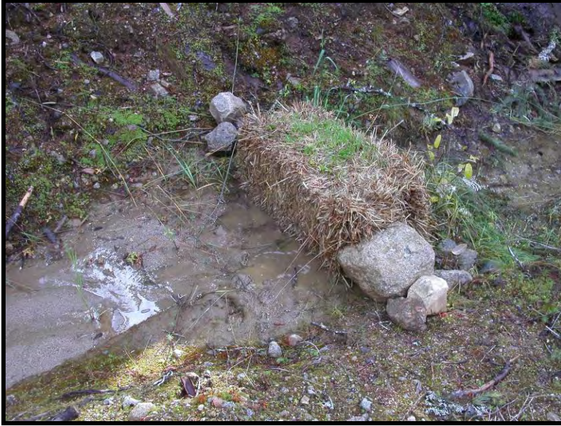
Figure 6. Straw bale placed in ditchline in Springer Creek. It is partially effective in blocking sediment, but requires regular maintenance to maintain its function.
