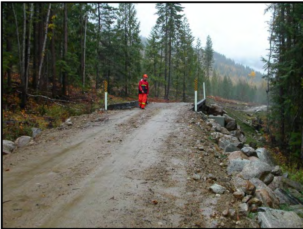
Figure 3. This bridge in Norns Creek is well aligned so that water drains away from the creek at both ends of the bridge. The bridge deck is also lined with geotextile material to help prevent dirt from getting into the creek.
