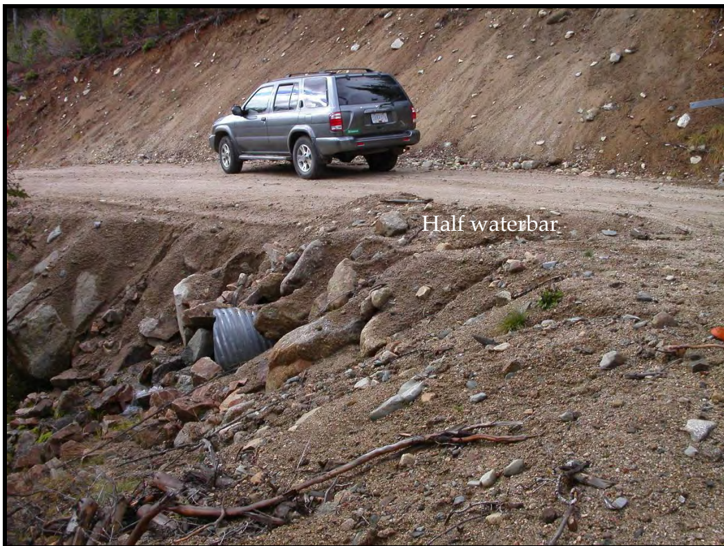
Figure 9. Half water bar installed above culvert in Springer Creek. The waterbar is not well placed since it directs water from the road near the culvert outlet, with direct connectivity to the creek. Where possible, road surface and ditch water that may transport sediment should be directed onto the forest floor. This site is also poorly vegetated.
