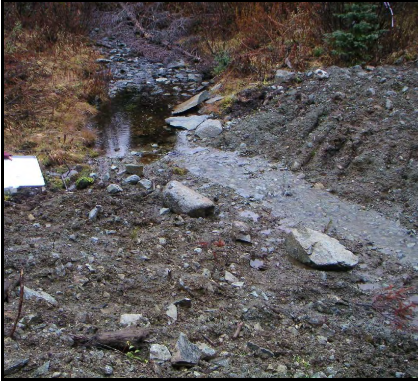
Figure 8. Deactivated road in Norns Creek. The natural drainage has been restored but the site has not been revegetated.
