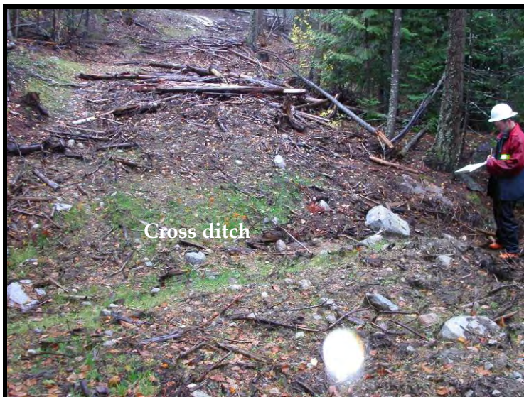
Figure 7. Deactivated road in Norns Creek. The road has been cross-ditched and is well vegetated at stream crossings.
