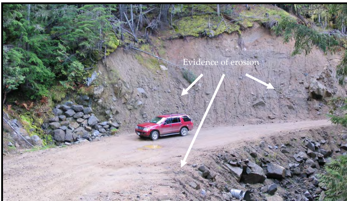
Figure 5. Large cutbank in Springer Creek. Large boulders have been placed near the culvert inlet as a stabilizing measure. Note the evidence of minor erosion on the cutbank and the road surface near the culvert outlet.
