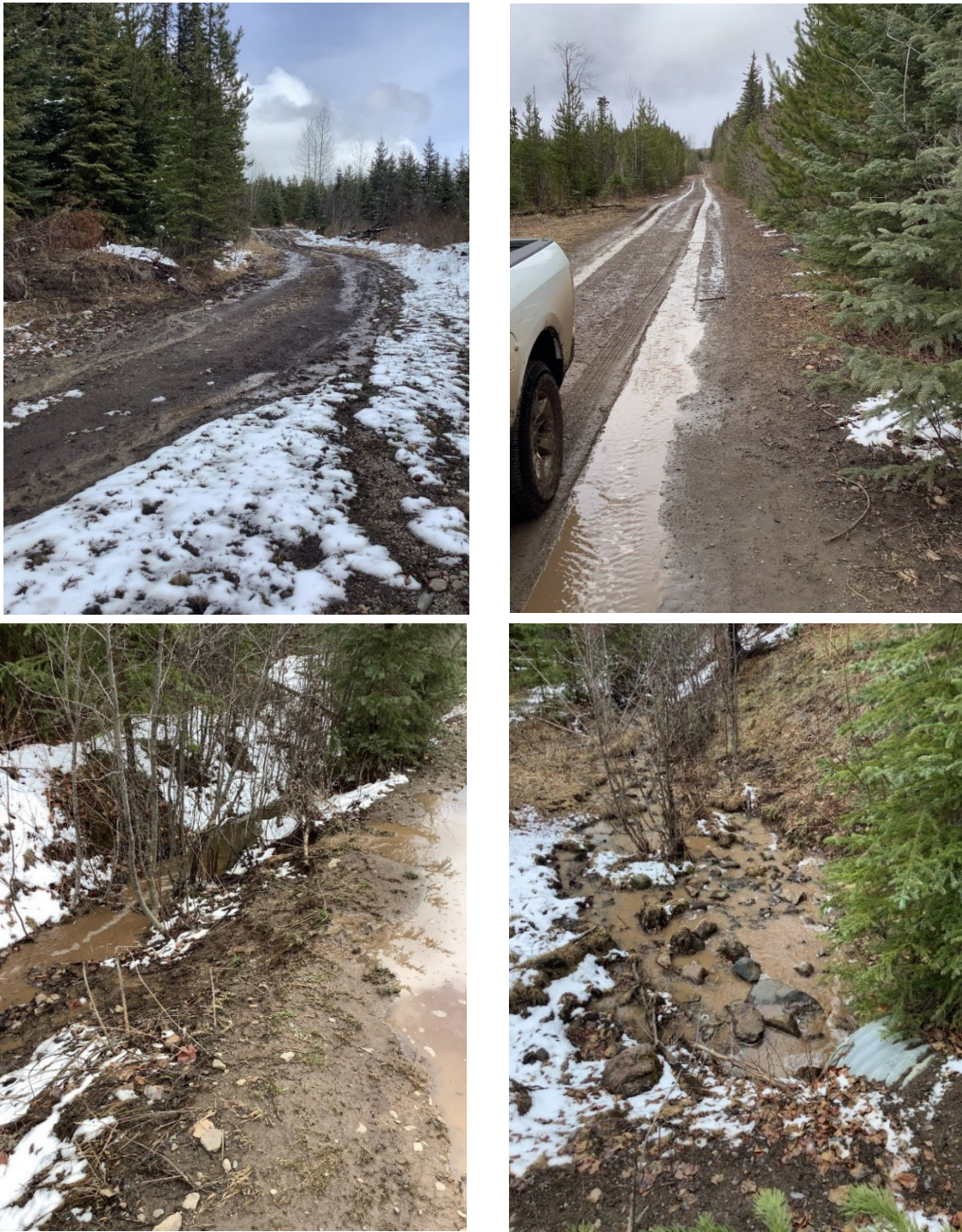
Figure 5. Water running down the surface of a W0104 road onto the mainline and draining into a tributary of Gardner Creek.
